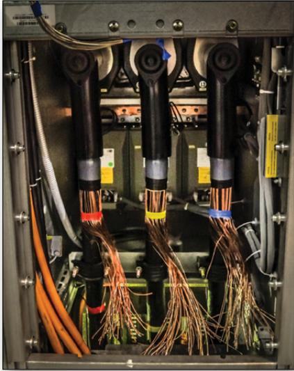
PBA's Tom Bromfield was engaged to provide training and supervision to the Fiji Electricity Authority (FEA) in Fiji's capital, Suva. FEA were replacing a 33kV switchboard and Tom provided training and supervision for the installation of the 33kV cable assets. FEA had not previously had any exposure to or formal training on 33kV elbow type termination plugs.
